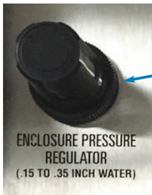
Figure F-14 Enclosure Pressure Regulator – Turn Clockwise
