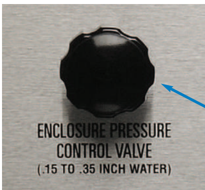
Figure F-16 Enclosure Pressure Control Valve
