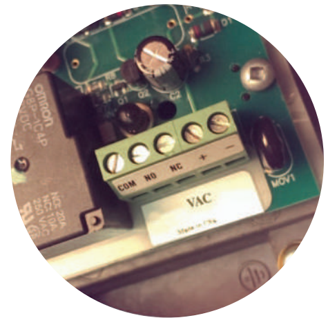
Figure R-7 DP-1C and DP-1D Terminal Block
